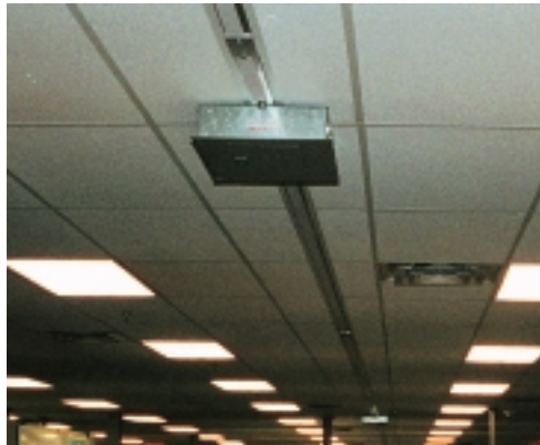
Engineering lab with Starline Track Busway recessed in ceiling over its workbenches and tables.
